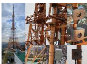
Namsan KBS Transmission Tower in Seoul (Dec. 2023 – Mar. 2024)
